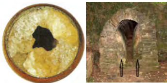
Figure 2.3.3: Calcium carbonate deposits (left) Calcium carbonate ( \text{CaCO}_3 ) deposits in hot water pipes can significantly reduce pipe capacity. These deposits, called boiler scale, form when dissolved \text{CO}_2 is driven into the gas phase at high temperatures. (right) Highly calcified remains of Eifel aqueduct near Euskirchen-Kreuzweggarten, Germany. (Wikipedia)
